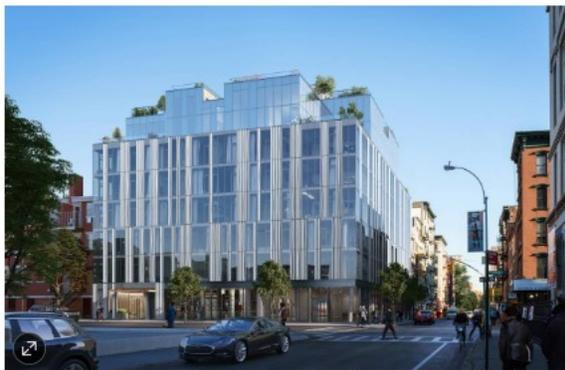
Rendering of 150 Rivington, a seven-story building with glass walls divided by cast-fiberglass panels, built on the site of a former matzo factory in Manhattan's Lower East Side neighborhood. PHOTO: VOLLEY STUDIO
